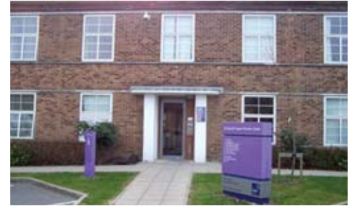
The current IAB HQ is located at Churchill Square, Kings Hill, near the Kent town of West Malling
